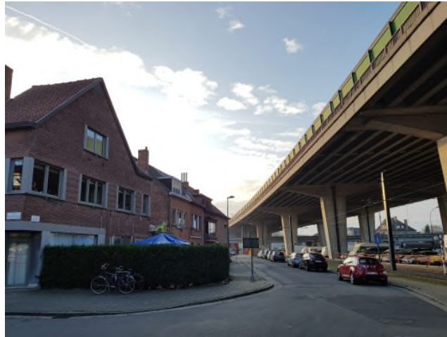
Figure 1. Highway viaduct cutting through a residential neighbourhood in Ghent, Belgium.
